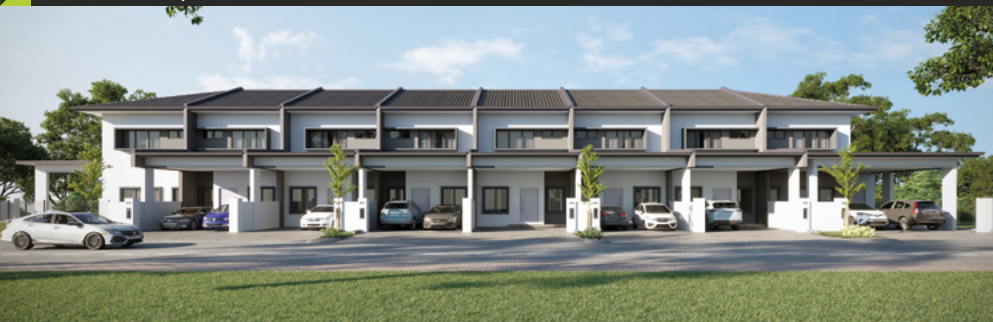
Our double storey terrace.
