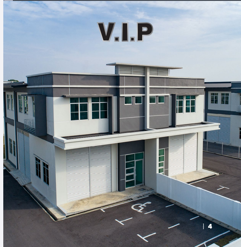
Built for heavy vehicles with XL size openings and high ceilings.
